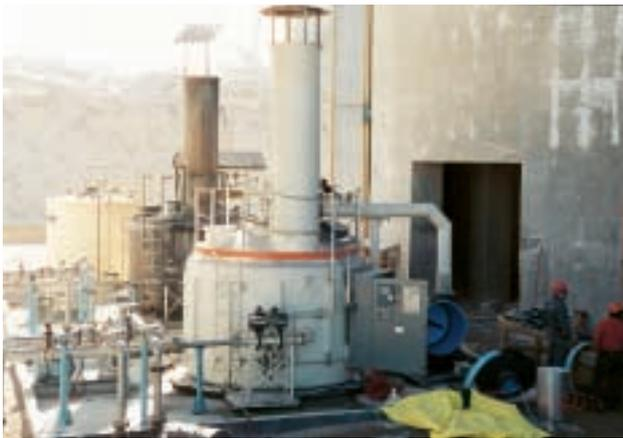
**Top:** 10 MM BTU/hr system for Rio Algom is used to heat the raffinate solution in a copper leach operation in northern Chile. **Middle:** 14 MM BTU/hr system for Ainsworth Lumber in Lillooet heats the recycle water used to condition timber blocks prior to veneer production. **Bottom:** 6 MM BTU/hr system for the Cameco uranium mine in northern Saskatchewan is used to prevent effluent ponds from freezing in winter.
